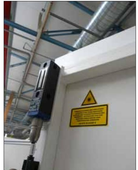
**Image 5 (sijenoptik 11):** The MZM 100 non-contact solenoid interlock is also used on the Jenoptik plants.
