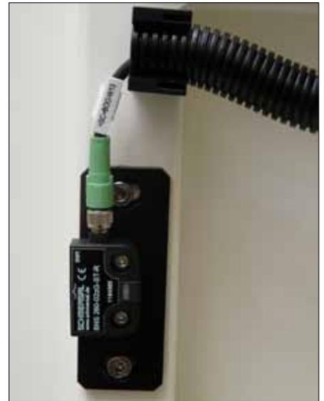
**Image 7 (sijenoptik 13):** When the laser plants are loaded, the safety sensors of the BNS 260 type retrieve the position of the pneumatically-powered bulkheads.
